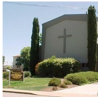
Walnut Creek United Methodist Church
